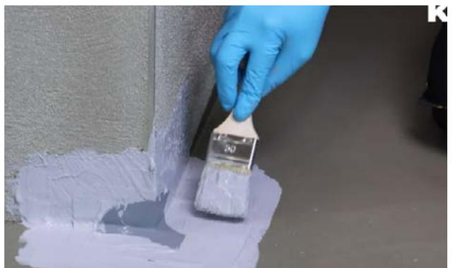
Alternatively, you can reinforce outside corners using a tailored piece of the KÖSTER Superfleece. In this case, two pieces are required: a strip measuring approx. 20 cm in length and a square piece roughly 10 x 10 cm. Fold this fabric strip in the middle and make a centered cut halfway through. Similarly, fold the square piece into a triangle and
