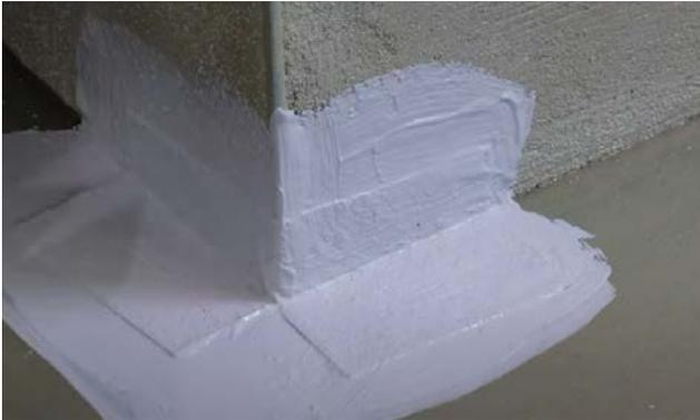
cut it halfway through as well. Embed the strip of KÖSTER Superfleece into the still fresh layer of KÖSTER BD 50, ensuring comprehensive coverage with KÖSTER BD 50. As for the square piece, place it with the cut side facing upwards and cover it with an additional layer of KÖSTER BD 50.
