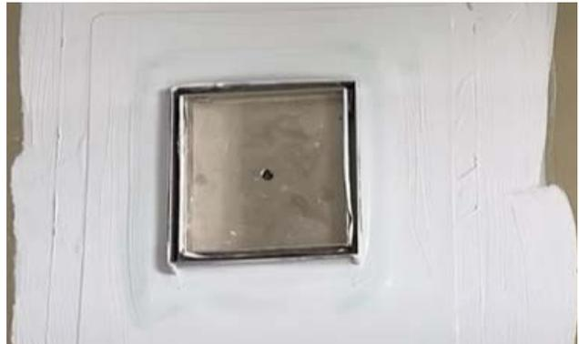
As an Alternative, a floor sleeve can be made using the KÖSTER Superfleece around the installed floor drain. The tailored cut piece is embedded in the pre applied layer of KÖSTER BD 50. After this, completely overwork the KÖSTER Superfleece with an additional layer of KÖSTER BD 50.
