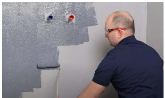
KÖSTER BD 50 is applied to the entire on the wall and floor surface using a roller or a brush. To minimize disruption and ensure a flawless application, it is recommended to begin by waterproofing all the walls and conclude with the floor areas.
