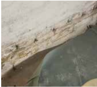
2. packer holes drilled
